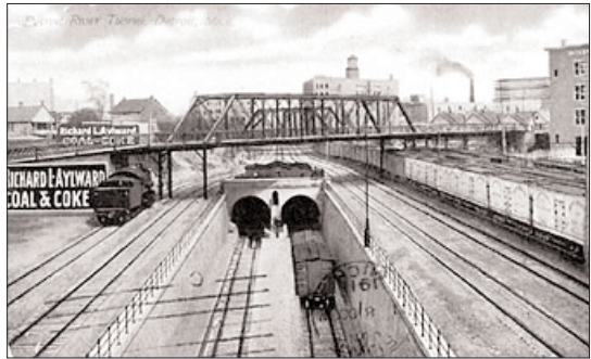
Windsor Detroit Train Tunnel 1912
